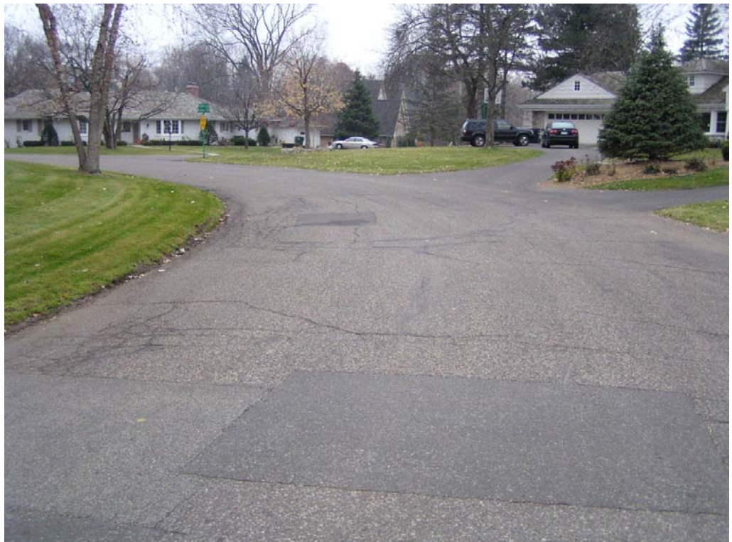
Photo 1. Existing Pavement Condition
